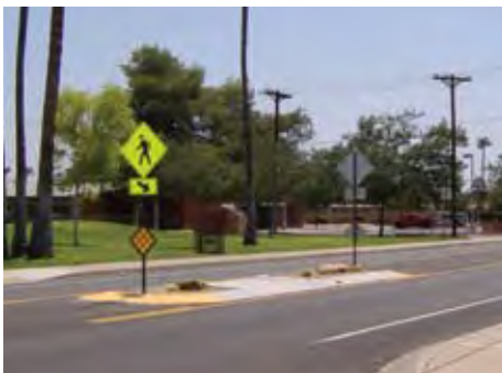
In-Street Pedestrian Crossing Signs
