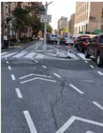
Intersection Crossing Markings
