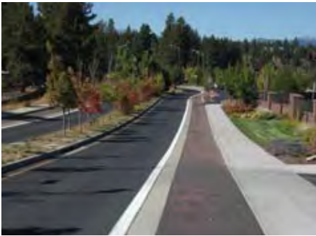
Raised Bike Lane
